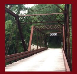
The Bridge: Motor Mill's current bridge, completed in 2012, is a replica of the pin-and-truss bridge which was built in 1899. In 1991 a flood took out one half of the original bridge. In 2008 another flood took out the remaining half. The total cost of the bridge project was estimated to be around \$1,000,000.
